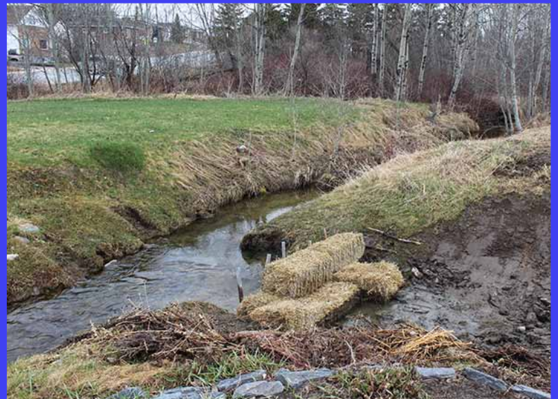
Town Creek maintenance work
