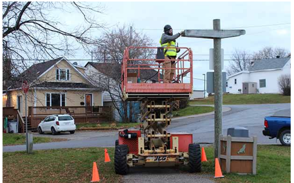
New LED lights were installed around Gillies Lake.
